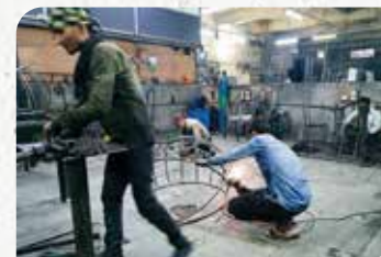
Metal CO2 Welding & Grinding
